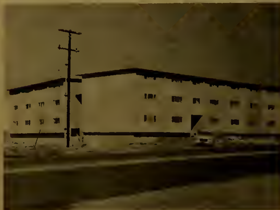
New McAfee Apartments NEAR completion.
